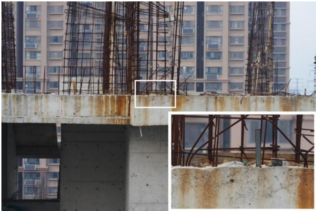
Construction Site 15m
