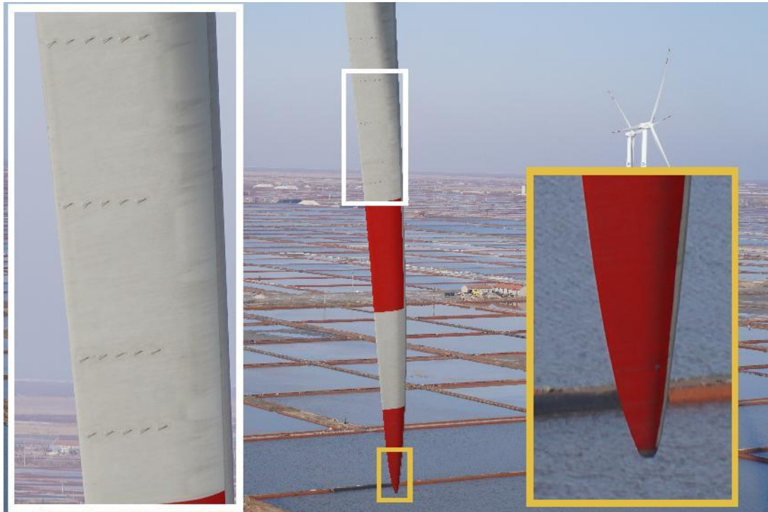
Wind-driven generator's blades inspection
